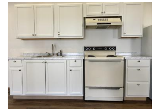
New Cabinets, Countertops and Sink
